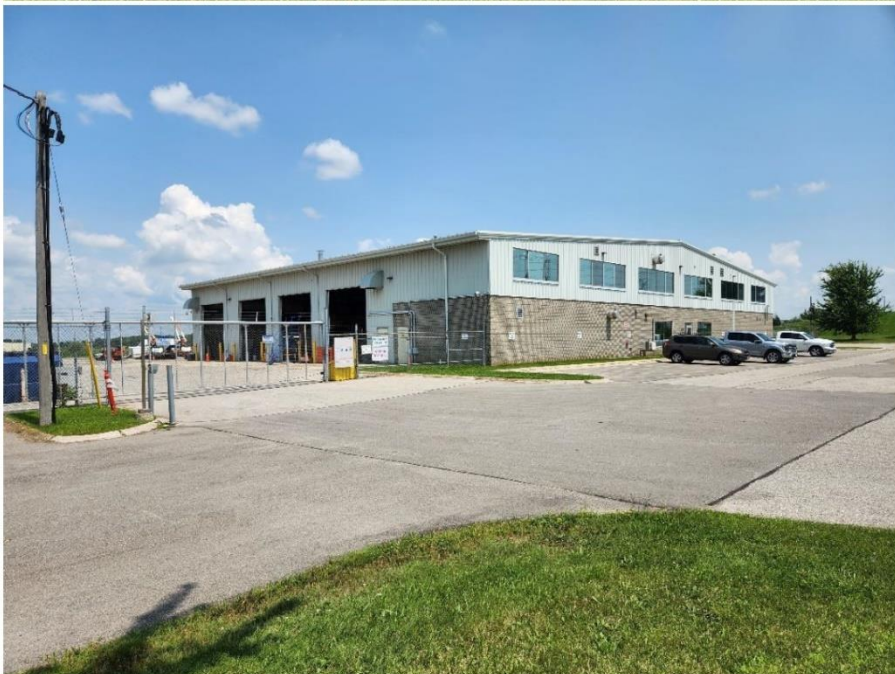
Hydro One Fleet Maintenance Services Facility
